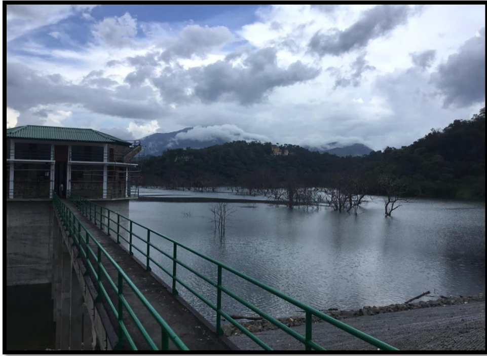
Dam of the Alikota Ara Reservoir
