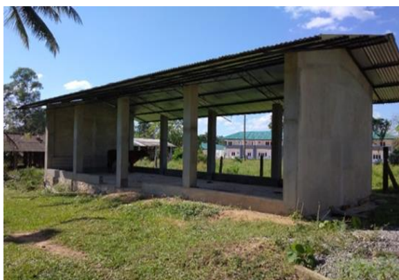
Chicken coop as at the date of inspection on 13 January 2020
