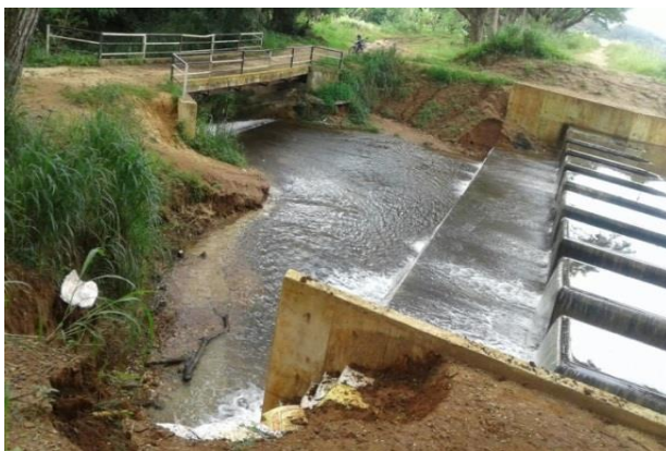
The bridge smaller than the spillway and insecure bank had been washed away by spill water
