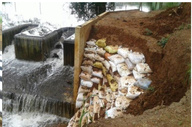
The bridge smaller than the spillway and insecure bank had been washed away by spill water
